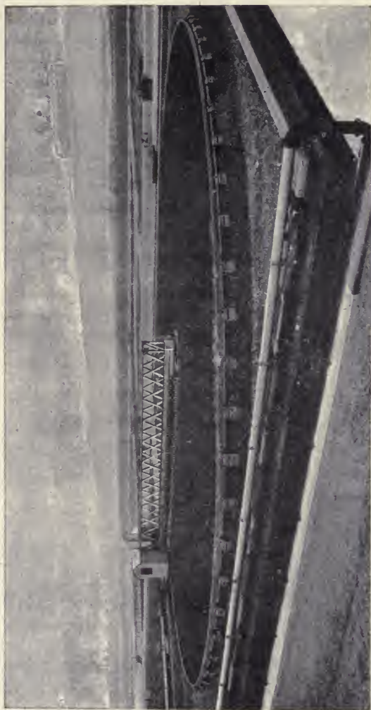
Fig. 17. Scott-Moncrieff's Effluent Distributor.
